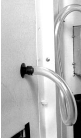
Figure 4: Back view of fascia
